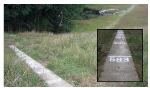
Construction wrapped up on repairs to four State flood control reservoirs in Stafford. In addition to the surveys and design of the repairs, Meehan & Goodin determined and painted the ground elevations onto a concrete flood stage guide along the upstream face of one of the dams, so that during a heavy rainfall, an observer will be able to determine the flood pool elevation from the top of the dam.
