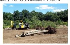
Shown above are the log "rootwads" queued on the banks. The photo below shows a section of the streambank with the first logs installed and the beginning of a "J-vane" in the distance.
